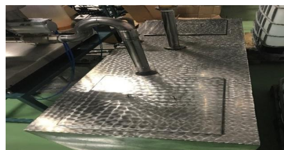
Figure 12 – Main Water Tank
