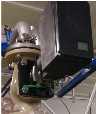
Figure 19 - Regulator Valves - Figure 20
